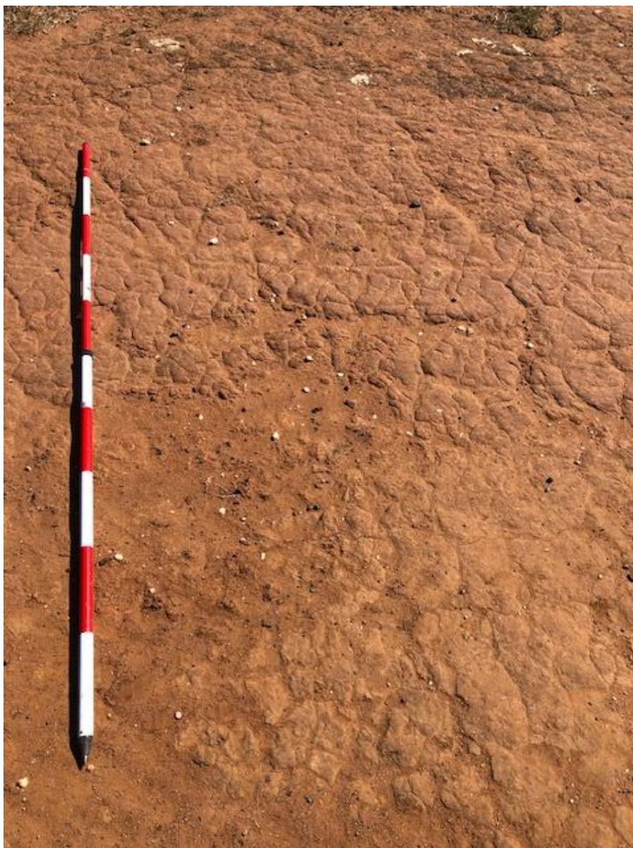
Plate 3. Example of hard baked surface scald road surface within Area 1.
