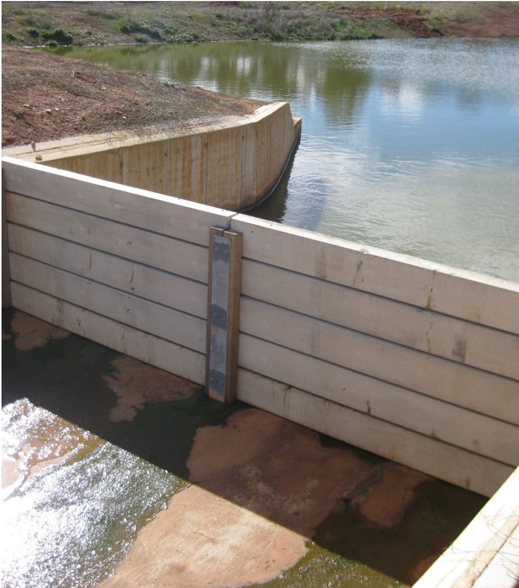
Photograph 12 – Sedimentation basin horizontal slat control outlet weir
